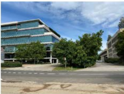
Picture 5 Entry points to 16 and 18 Lexington Dr. looking south east of the site
